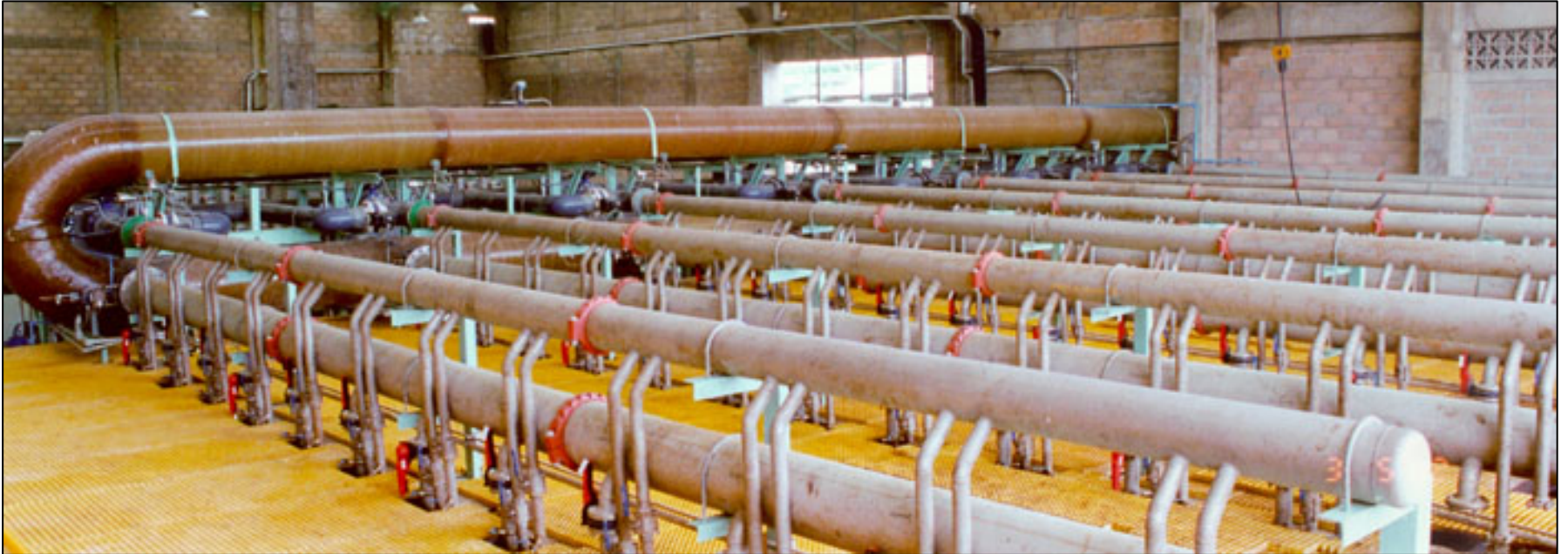
UF membrane process trains
