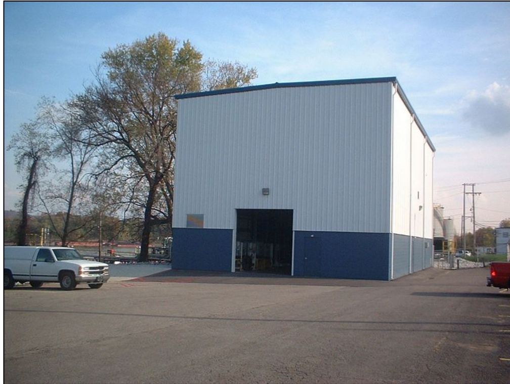
Membrane equipment building
