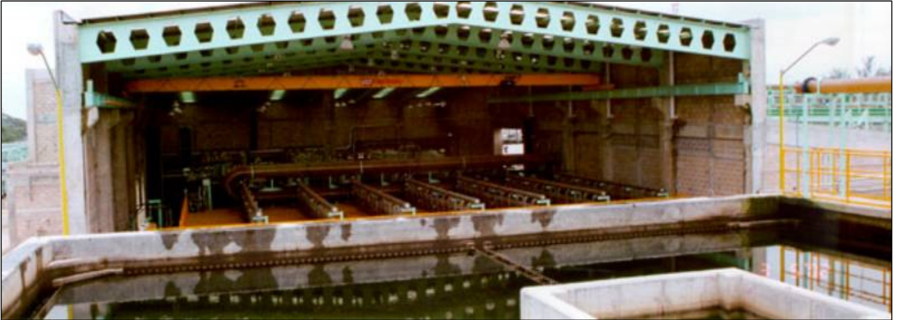
UF membrane process trains in treatment building
