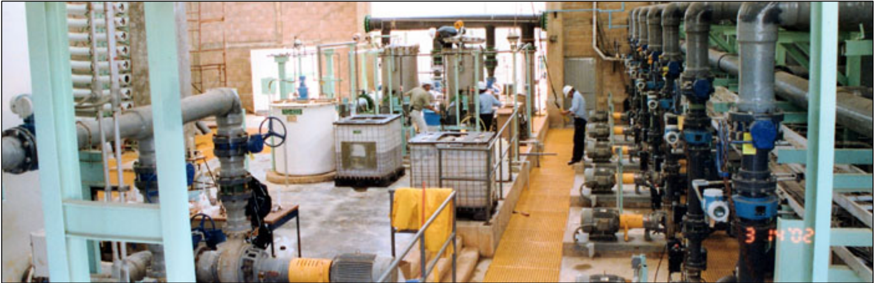
UF membrane process equipment
