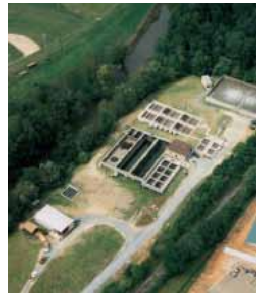
The basins of the Vertical Loop Reactor system share common walls, reducing construction costs.
