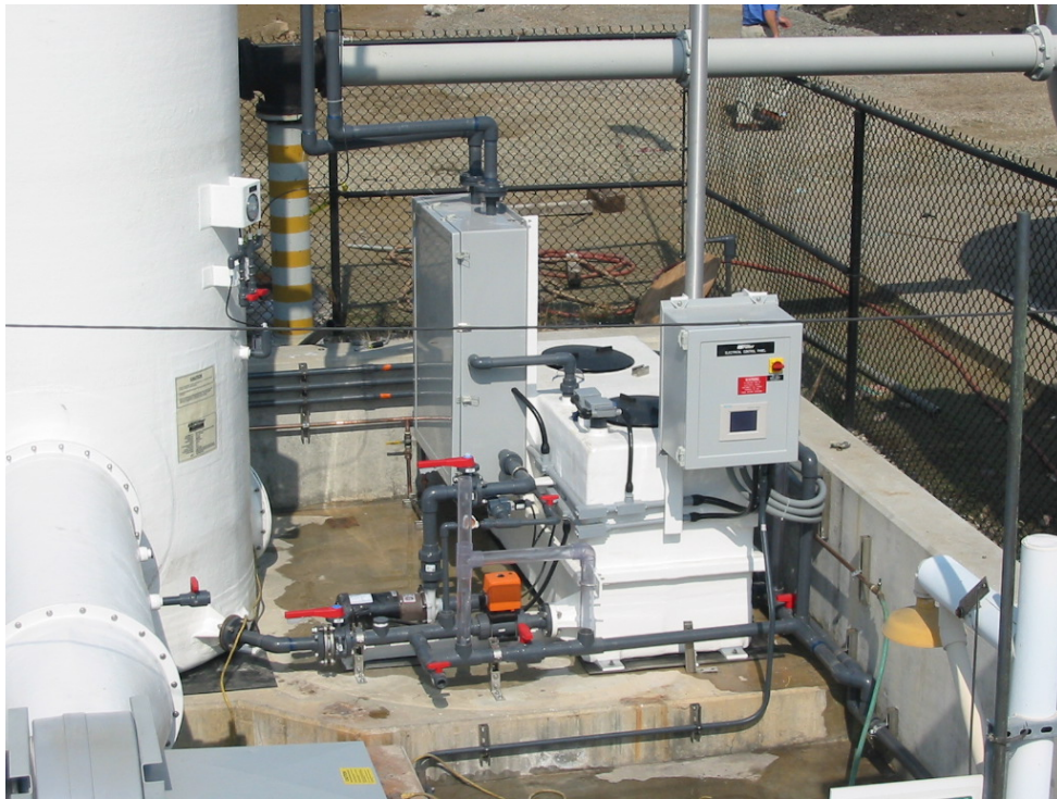
Figure 6 shows the ZABOCS BTF “Nucirc” skid assembly.
