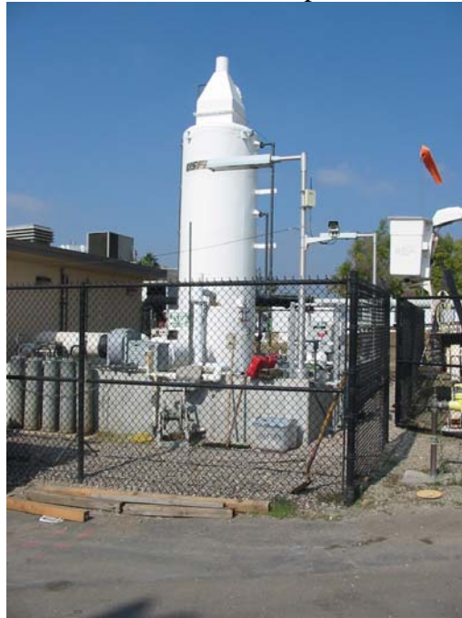
Figure 2: Biotrickling filter odor control system at Influent Pumping Station
