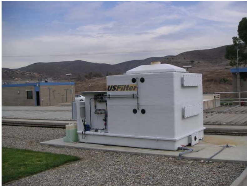
Figure 3. ZABOCS Biofilter at Padre Dam WRF.
