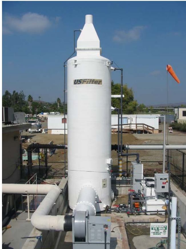
Figure 4. ZABOCS BTF Bio-tower at Padre Dam WRF.
