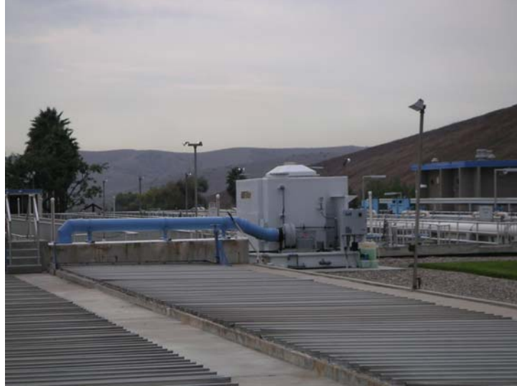
Figure 1. ZABOCS Biofilter at Padre Dam Water Reclamation Facility
