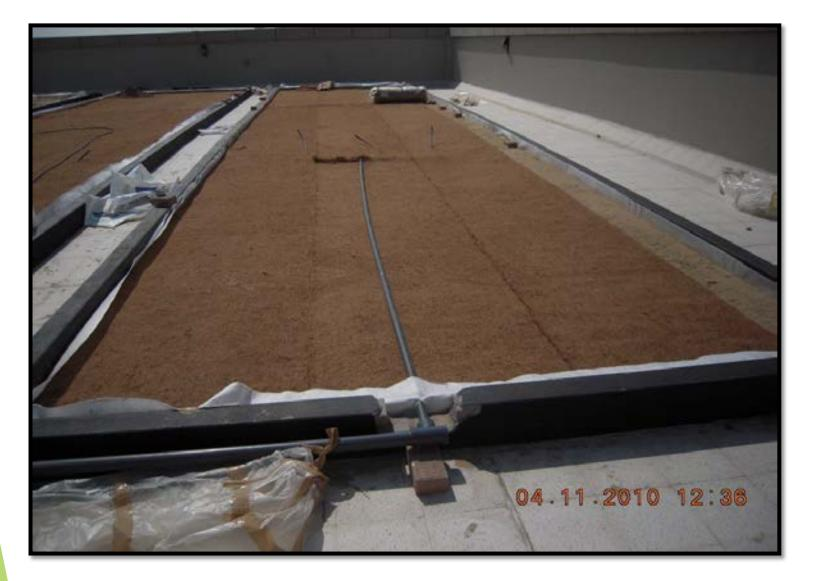
Two layers of Green Mat are spread on top of the drainage layer with growing media in between. Irrigation pipes are also installed.
