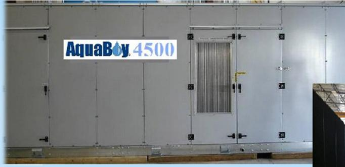
18,000 liters per day Can reclaim R/O water-25% 200 tons of cold A/C Pure Water From Air
