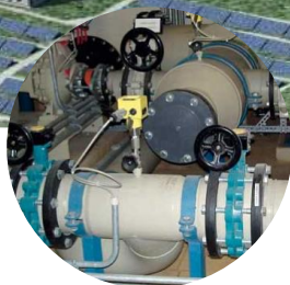
Flue Gas Desulfurization
