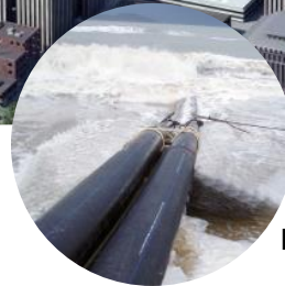
Water Intake Lines
