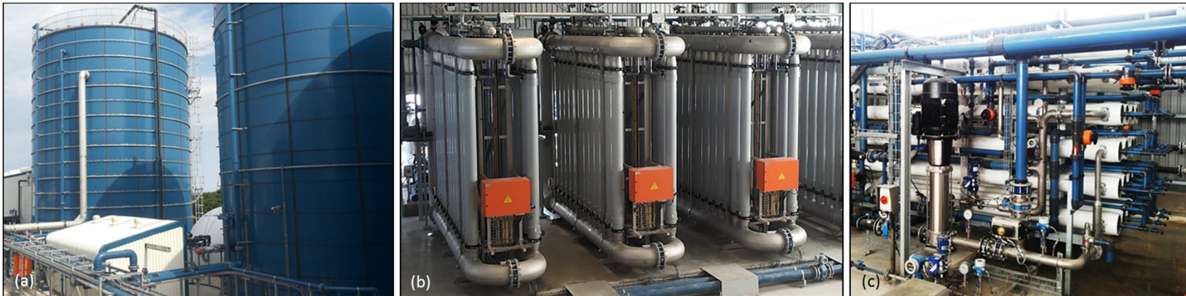
AnMBR + RO full-scale plant at Site 1: (a) Buffer tank & Digester; (b) AnMBR UF skids; (c) RO
