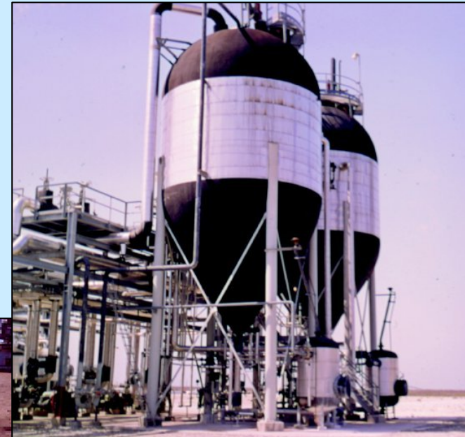
Hot Lime Softener - Silica Removal for Boiler Feed Water
