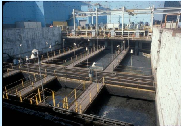
Oil Removal w/ Mill Scale Collector and Oil Belt Skimmers Steel Mill
