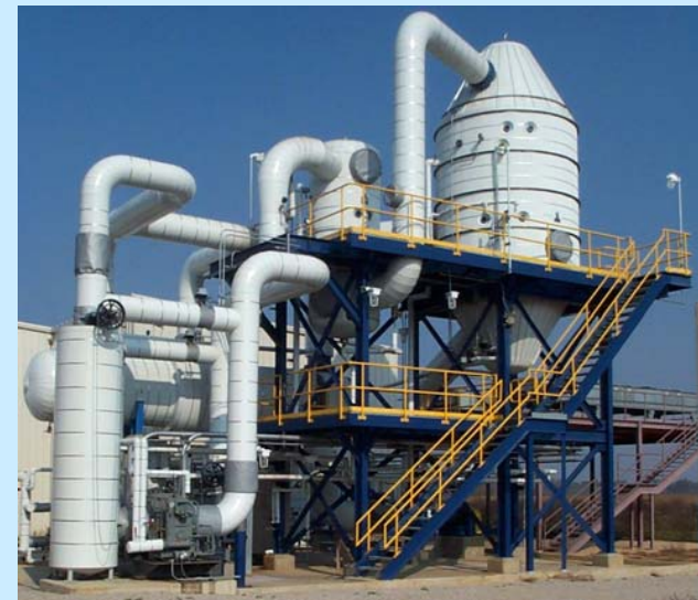
Brine Concentrator Chemical Plant
