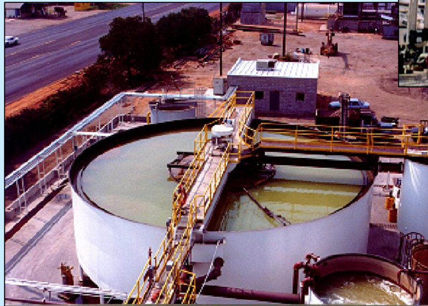
Solids Contact Clarifier – Metals Removal Pipe Mill
