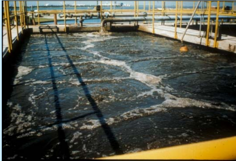
Fine Bubble Aeration – Paper Mill
