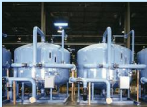
Industrial Process Water
